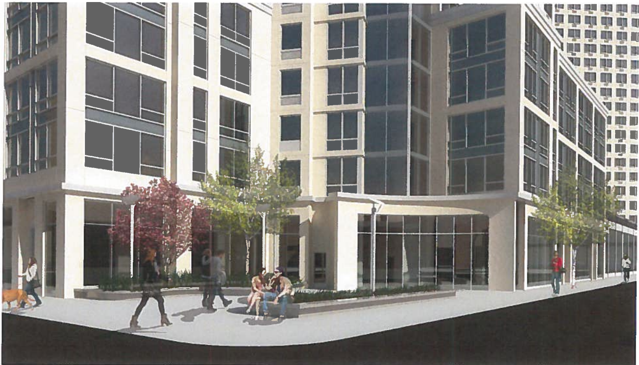
Entrance on Jackson Avenue
